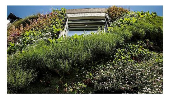
Retrofitting an existing masonry cavity walled building with a green or living wall can reduce the amount of heat lost through its structure by more than 30%, according to new research conducted by the University of Plymouth.
