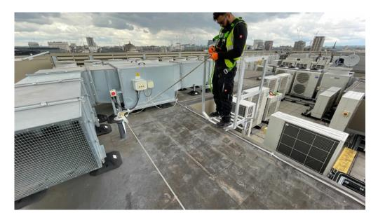
A team of specialist engineers from GIND UK is on site at a major refurbishment project at 30 Panton Street in Central London, where they are undertaking safety wire quality checking and testing of a new façade access system.
