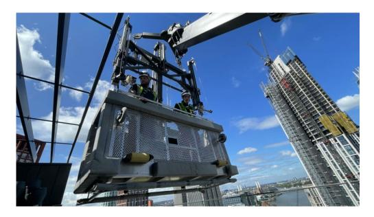
A team of specialist engineers from <u>GIND UK</u> is on site at Damac Tower, on London's South Bank, where they are undertaking final testing and commissioning works on the pantograph recessed façade system and green roof prior to handover of the project.
