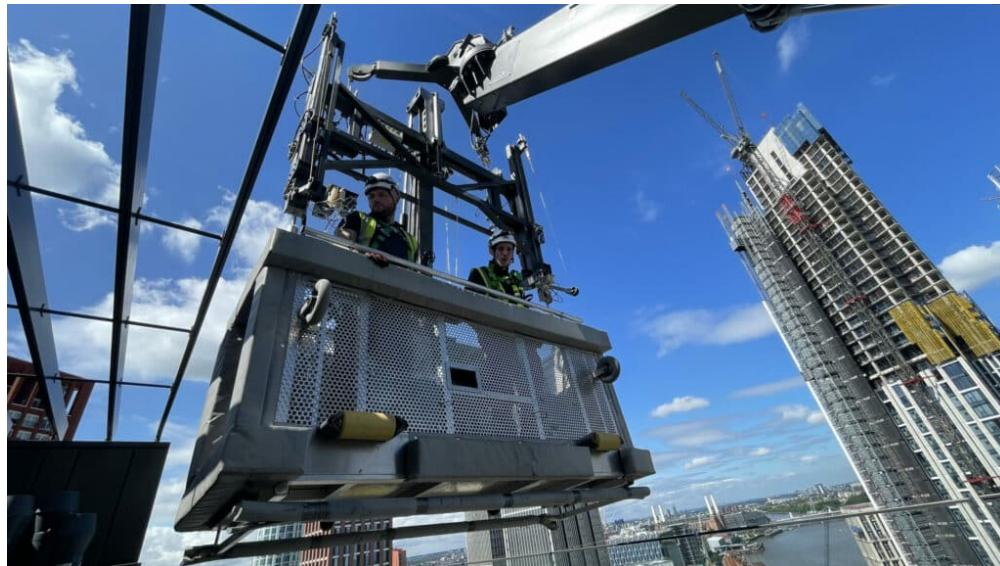
A team of specialist engineers from [GIND UK](#) is on site at Damac Tower, on London's South Bank, where they are undertaking final testing and commissioning works on the pantograph recessed façade system and green roof prior to handover of the project.
