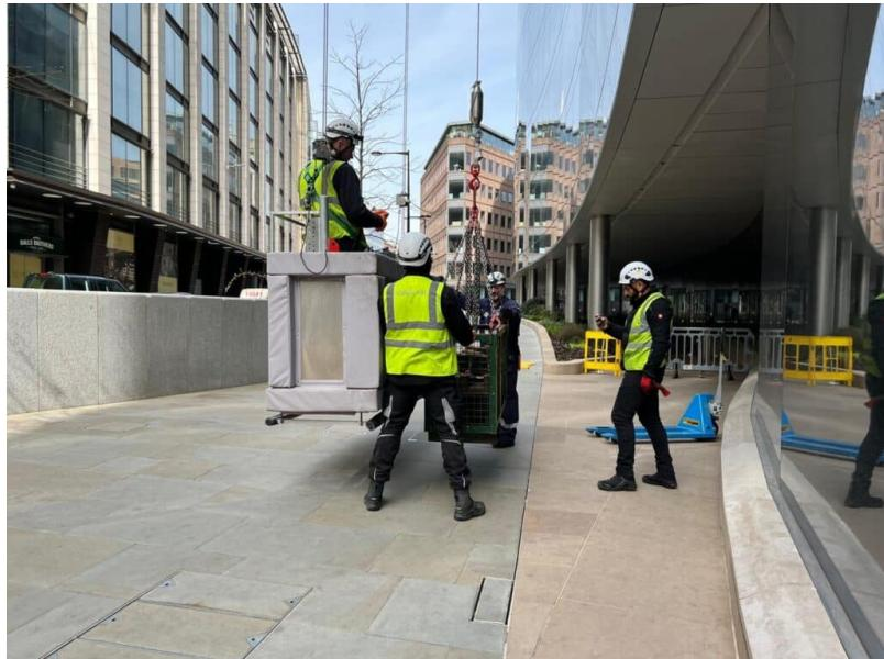
A team of specialist engineers from GIND UK is on site at Plumtree Court in London – the new headquarters of Goldman Sachs – where it is conducting quality and load testing of the building's façade access equipment.
