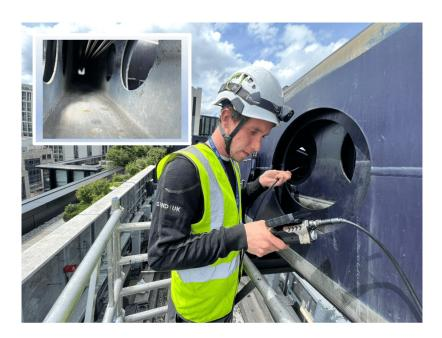
The maintenance team at <u>GIND UK</u> are using an endoscope to carry out inspections of the internal jib wires and mechanism as part of the BMU testing and commissioning works at 185 Park Street, London.
