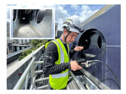
The maintenance team at <u>GIND UK</u> are using an endoscope to carry out inspections of the internal jib wires and mechanism as part of the BMU testing and commissioning works at 185 Park Street, London.
