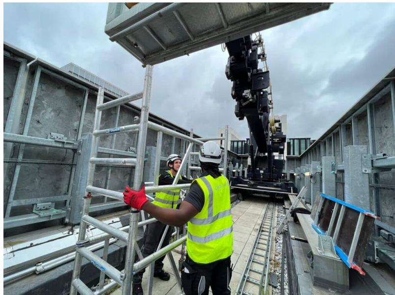
Following the successful and safe installation of a façade access solution comprising multiple BMUs at 185 Park Street, London by Integral Cradles, GIND UK starts the testing and commissioning process to get this technically challenging access equipment into warranted use.
