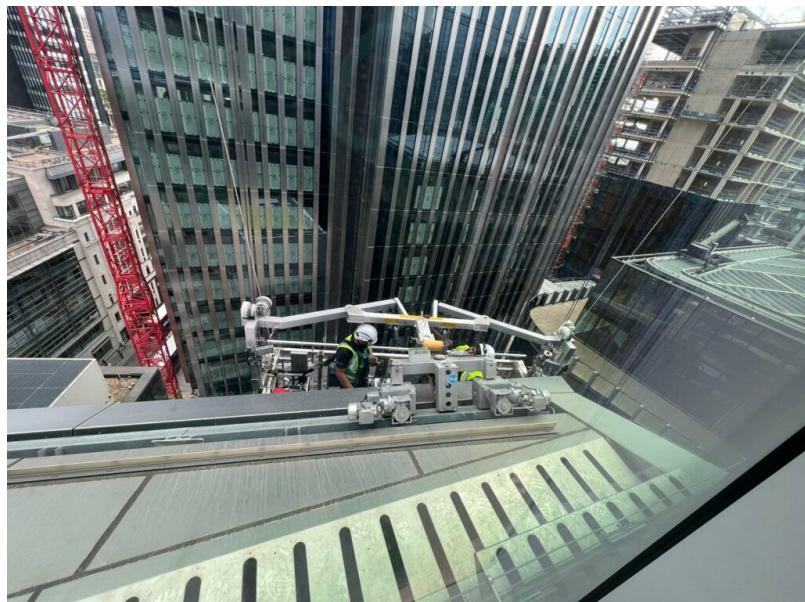
[GIND UK](#) is currently on site at 52 Lime Street (The Scalpel) to test the diverter trolley. The team are using the award-winning building maintenance unit (BMU) designed and installed by sister company Integral Cradles.
