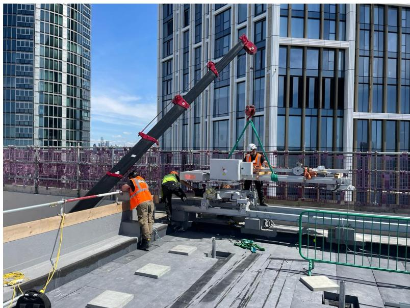
[Integral Cradles](#) has installed another high quality building maintenance unit (BMU), this time for MACE on the project One Thames City N6. Without the use of the tower crane, Integral Cradles successfully completed the installation with the use of its own spider crane, which was assembled and disassembled using the project hoist.
