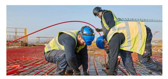
Building specifiers and contractors looking to tackle the increased risk of buildings overheating via Thermally Activated Building Structures (TABS) can now implement industry-leading smart technology for efficient heating and cooling.
