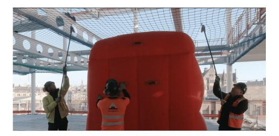
This solution means that an operative can be easily rescued in under three minutes, in spaces where the floor to height is as low as 3.5 metres.
