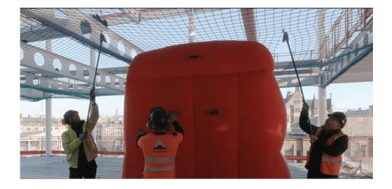
This solution means that an operative can be easily rescued in under three minutes, in spaces where the floor to height is as low as 3.5 metres.
