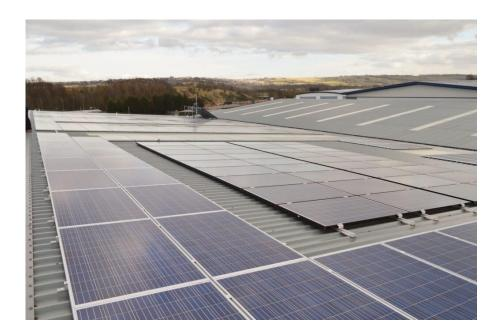
Custom Solar, part of <u>Mitie</u>, has completed the installation of a 1.25MWp roof-top solar PV array at Pets at Home's new National Distribution Centre in Staffordshire. The distribution centre, which opened in early 2024, supplies products to the pet care brand's 450-plus stores.
