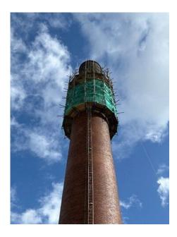
P<u>remier Technical Services Group Ltd</u> (PTSG) has begun work in Manchester, where its specialist steeplejacks are reducing the height of a disused brick chimney.
